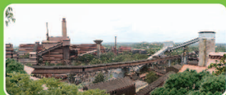
View of Pellet Plant
