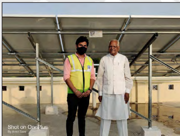
President of India Ram Nath Kovind (R) during inauguration of the solar plant...
