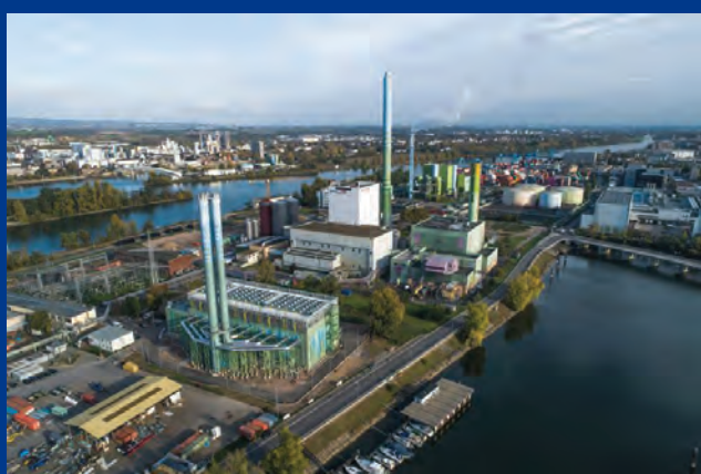
Aerial image of Kraftwerke Mainz-Wiesbaden AG power plant delivered by Wärtsilä... Image © Wärtsilä Corporation
