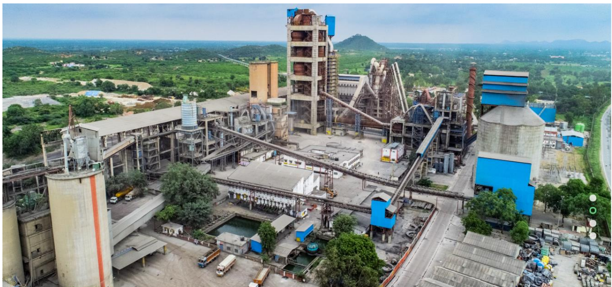
Figure 2.1 A view of UCWL's Integrated Cement Plant
