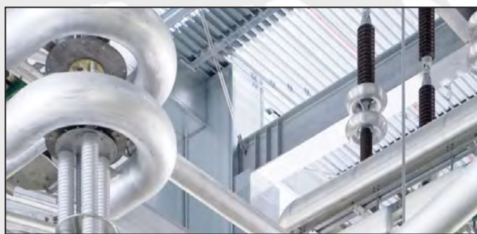
A view of a part of the project...
