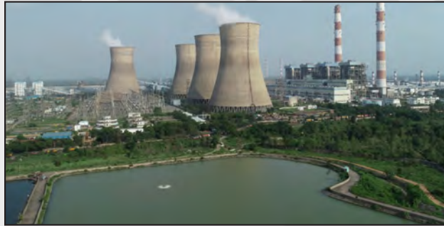
Vedanta's captive power plant at Jharsuguda, Odisha...
