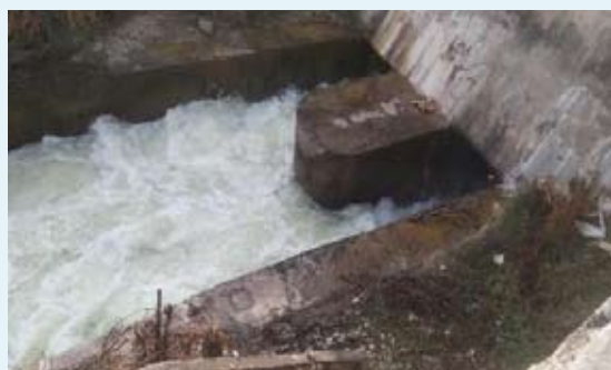
(c) Well type outlet Mashri Dam (Available head 4 m)
