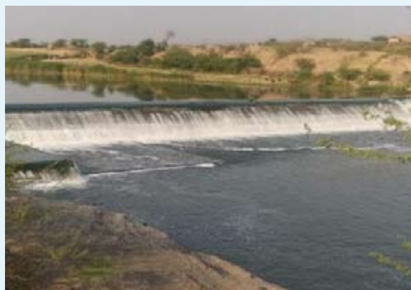
Fig. 5 : Check Dam on Mej River near Lakheri Town in Bundi District (Approximate head is 5 m)
