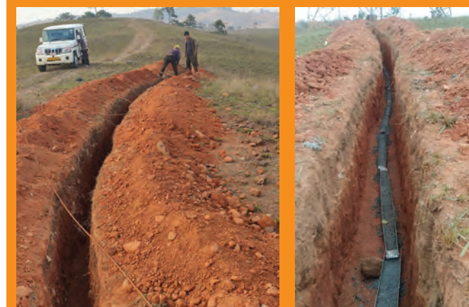
Marconite earthing execution work...
