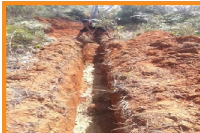
Bentonite application work...
