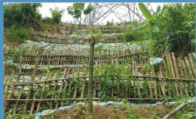
Fig: 3B - Temporary protection locations...
