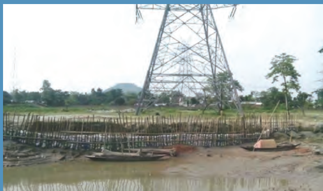
Fig: 4C: Temporary protection in old location...
