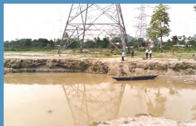
Fig: 4B: Anchor Tower in old location...
