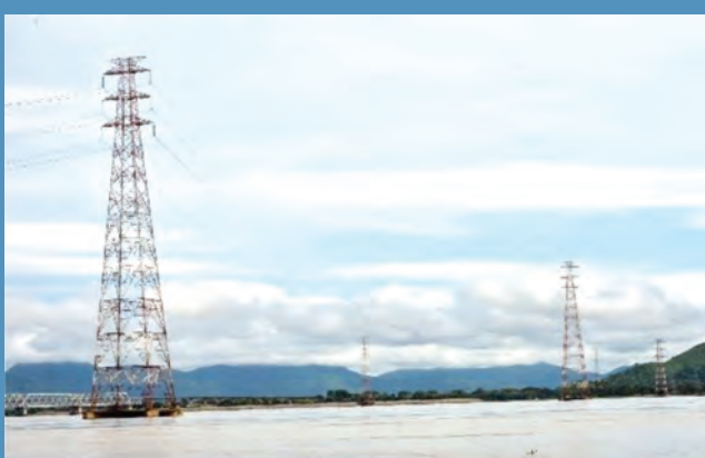
Fig: 4A: Two nos. well foundation locations...
