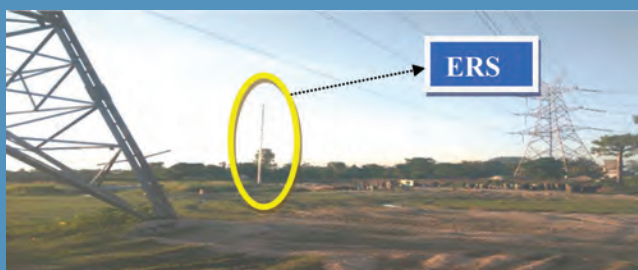
Fig 4D: Use of Emergency Restoration System (ERS)...
