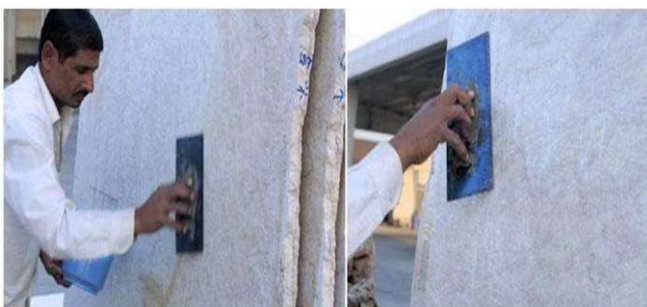
Figure 26. Net-reinforcement of Marble Slabs
