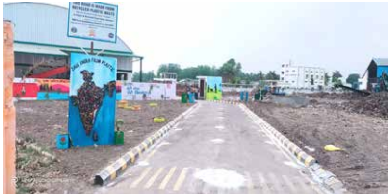
Road constructed using Plastic Waste at MRF Haridwar
