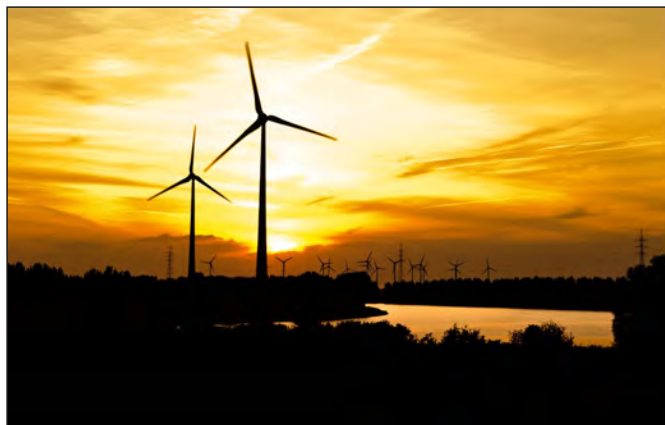
A glimpse of the RE power plant in Poland...
