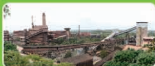
View of Pellet Plant
