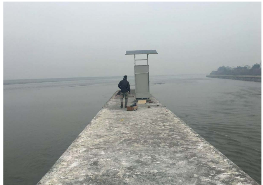
Madhya Ganga barrage
