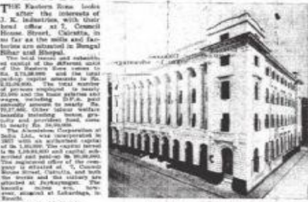
Eastern Zone Building in Calcutta.
