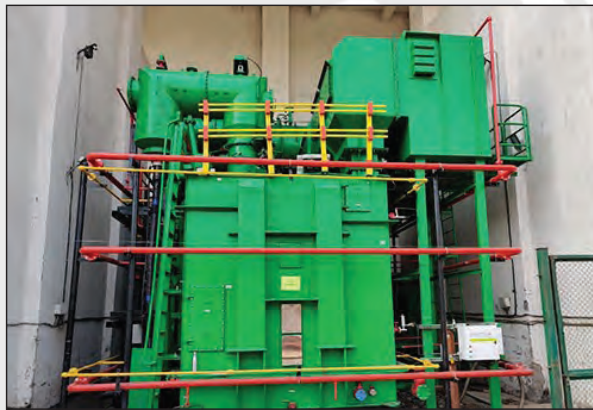
The natural esters used in these transformers have a high fire point (3500C)...
