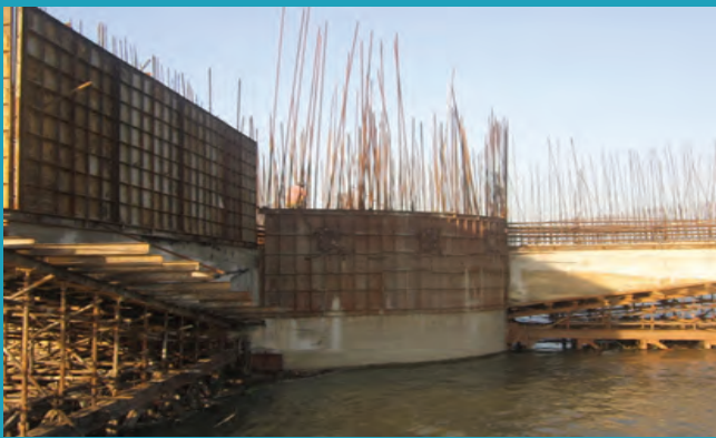
View showing Shuttering work for Cantilever beam portion...
