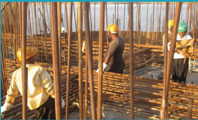
View showing – Reinforcement work of well cap 2nd stage is in progress...
