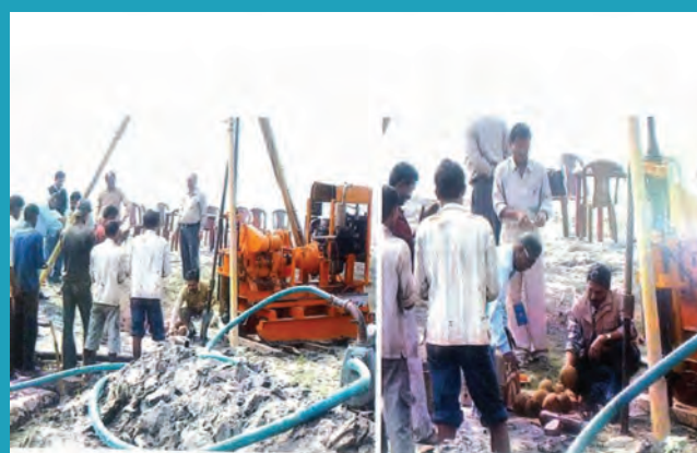
The piling work at the time of construction...
