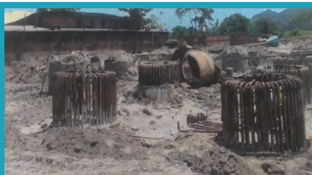
The steel structure at the time of construction...
