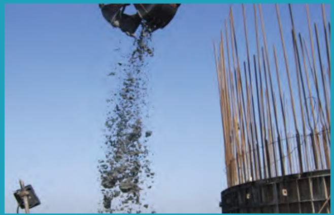
View showing –Sinking is in progress
