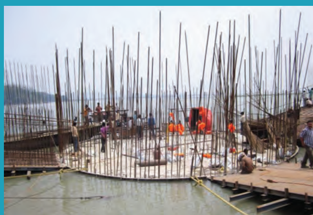
Photo 2: GPS view of well foundation on river Brahmaputra during construction phase...
