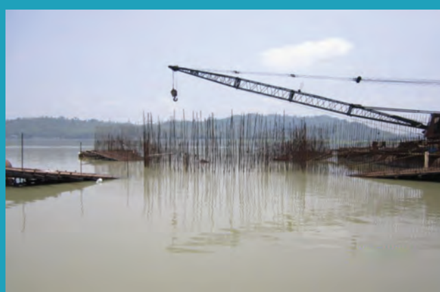
Photo 3: GPS view of well foundation on river Brahmaputra during construction phase...
