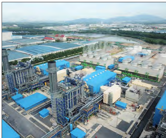
The GTCC Power Plant in Chonburi...
